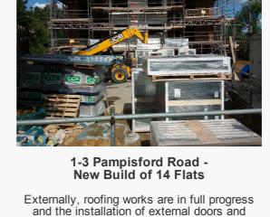
windows are nearing completion. Internally, Mechanical & Electrical first fix is complete, with plastering due to commence this month.
